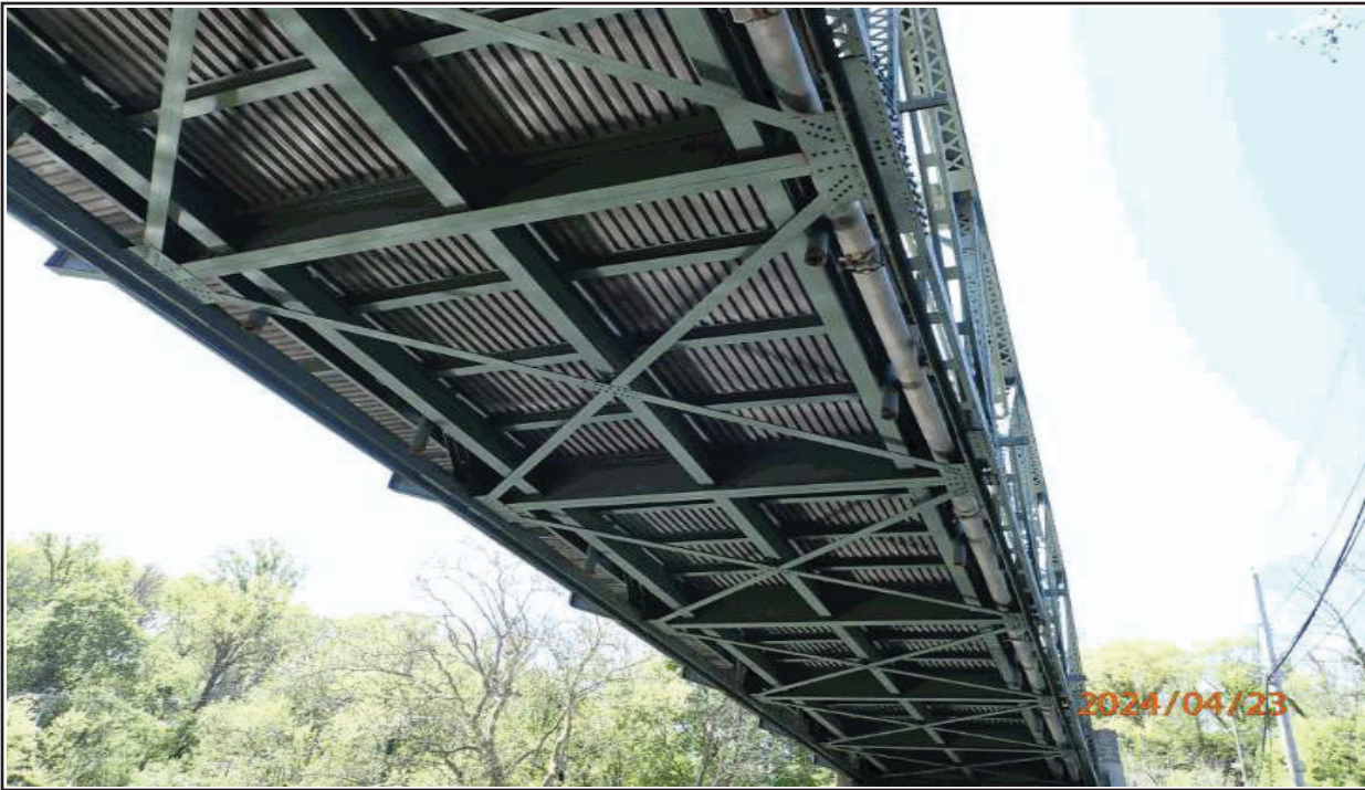
3 TYPICAL VIEW OF UNDERSIDE, LOOKING SOUTH
