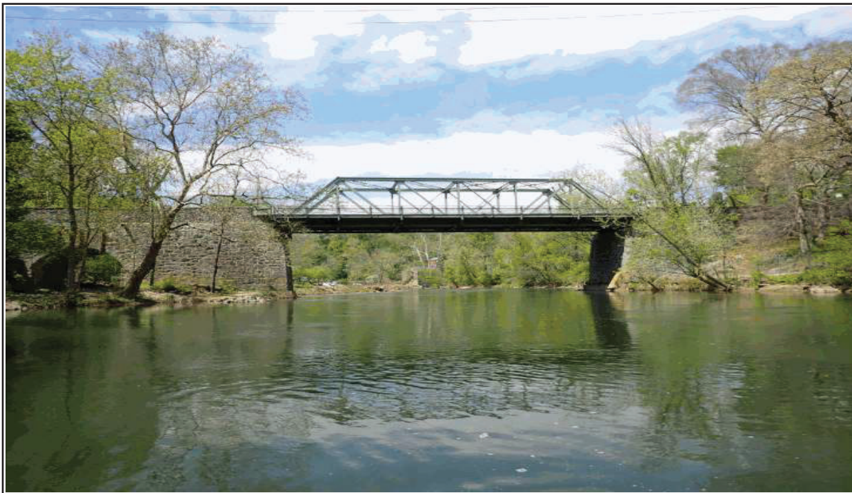
2 EAST ELEVATION LOOKING WEST
