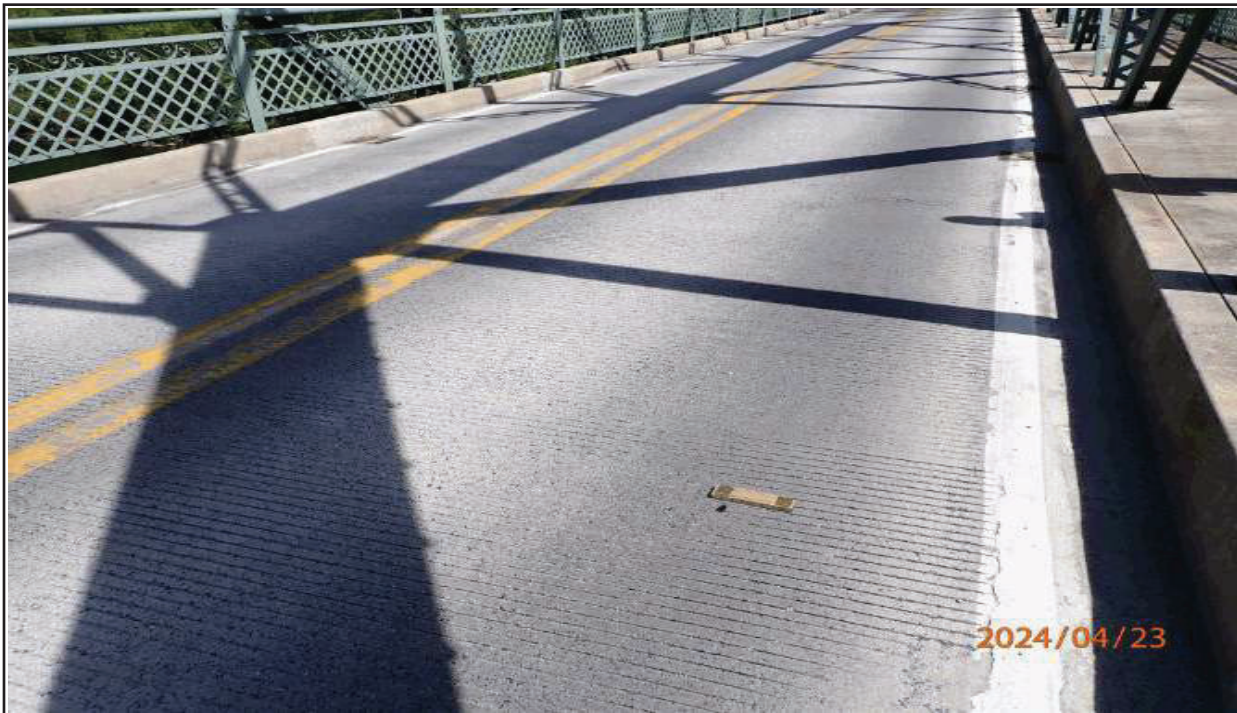
6 GENERAL VIEW OF DECK, LOOKING NORTH
