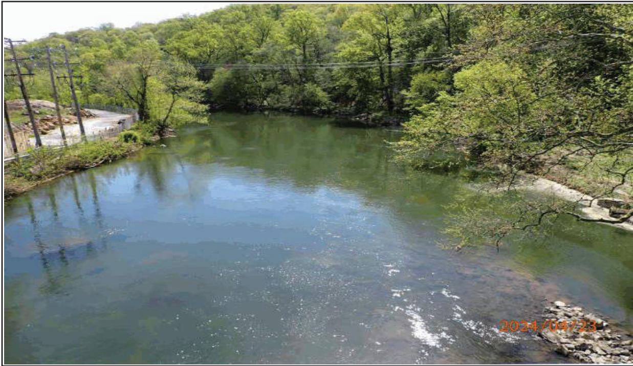
5 BRANDYWINE CREEK, LOOKING DOWNSTREAM (EAST)
