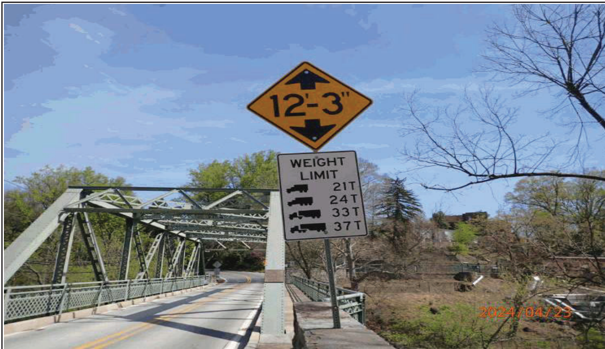
8 VERTICAL CLEARANCE AND LOAD POSTING SIGNS AT SE CORNER (NW SIMILAR)
