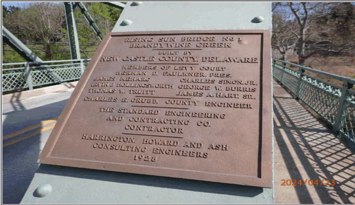
7 BRIDGE PLAQUE AT SOUTHEAST CORNER (NORTHWEST CORNER SIMILAR), LOOKING NORTH
